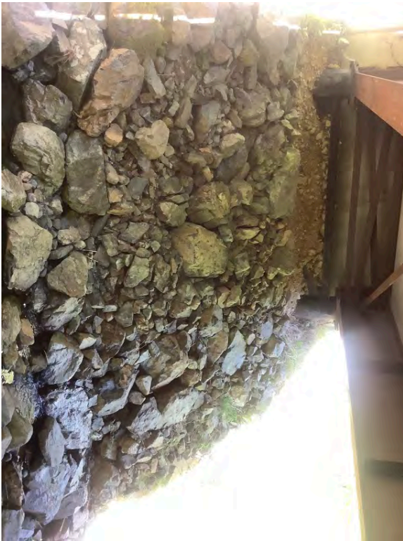
Left Bank Abutment when facing downstream
